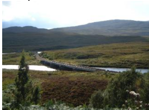
Railway viaduct at eastern end of site
