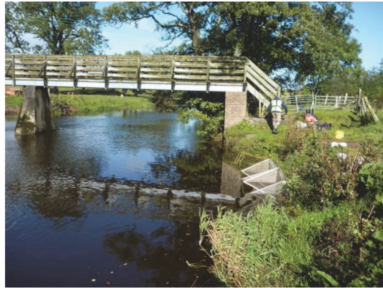
Site E12 from downstream
