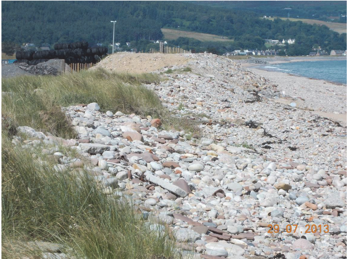
Figure 6: The Kart Track embankment lies 2m vertically above the height of the adjacent coastal edge to the south.
