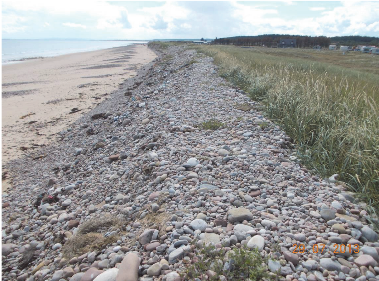
Figure 5: Reprofiled coastal ridge at the caravan park and lower land to the rear.
