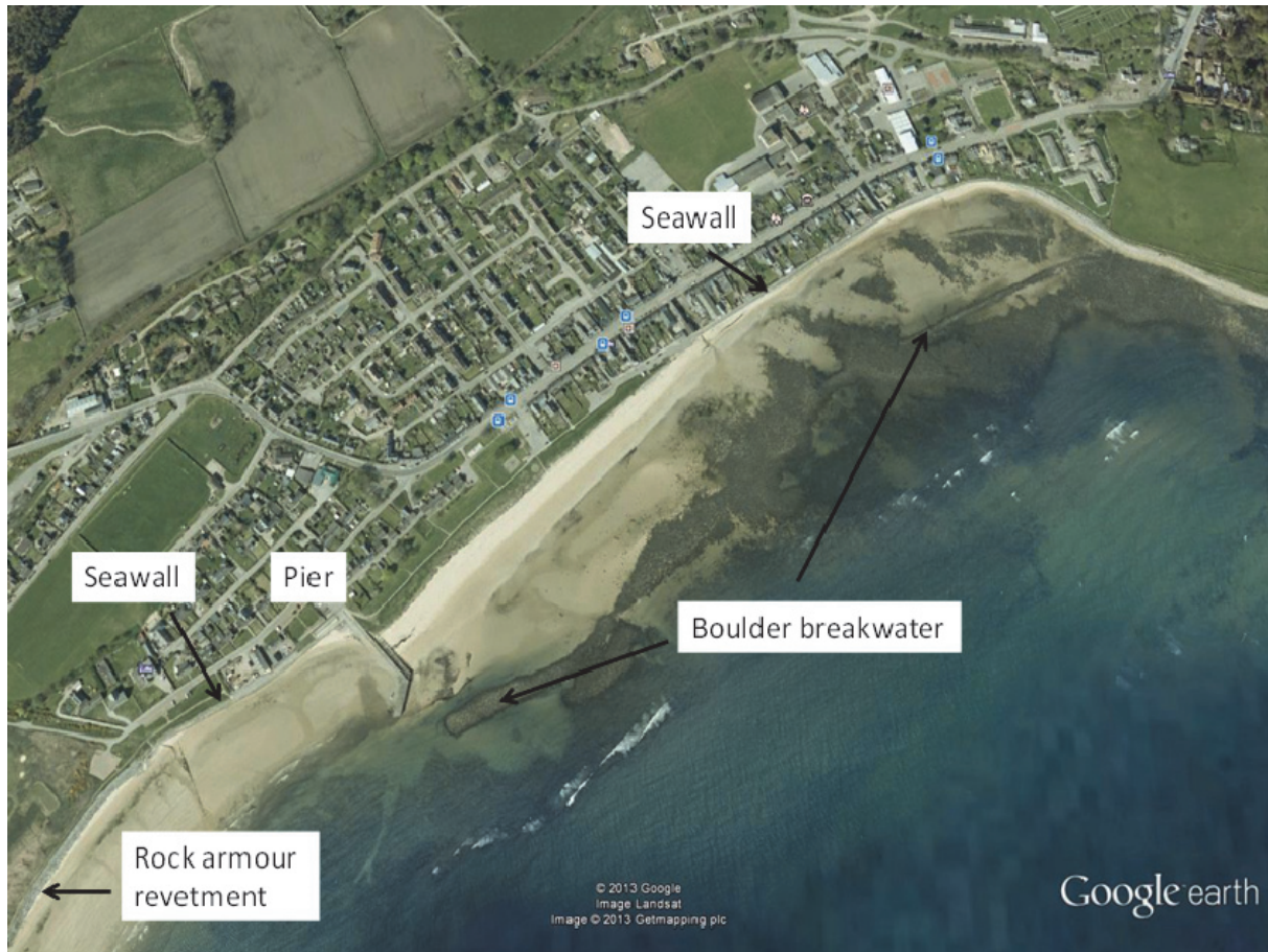
Figure 3: Golspie seawalls, pier and breakwater fronting the town and rock armour revetment fronting the northern part of the golf course.
