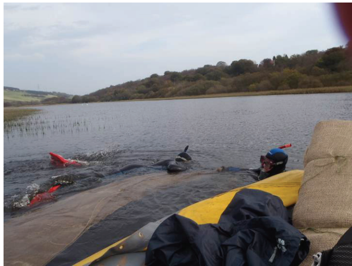
Divers towing jute matting out to required position from inflatable boat (2011)
