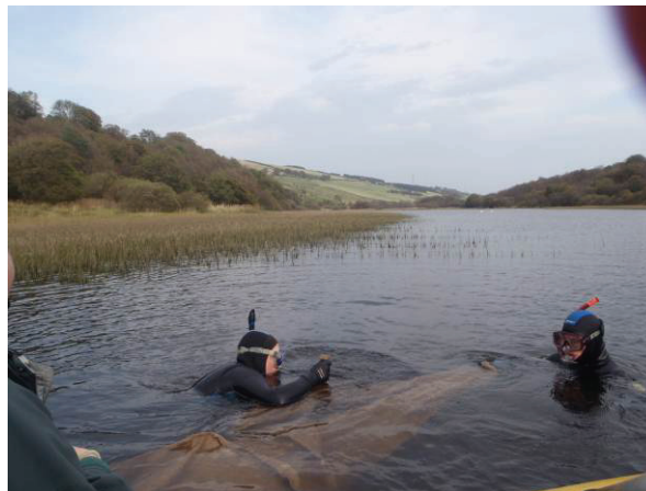
Figure 4.2: Snorkel team installing the jute matting
