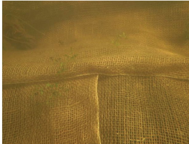
Figure 4.4: Overlap between adjoining sheets of jute matting
