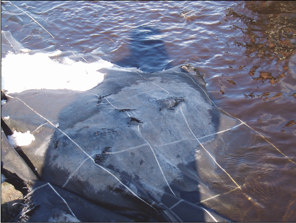
Plate 11. Weed control fabric fraying due to contact with rocks
