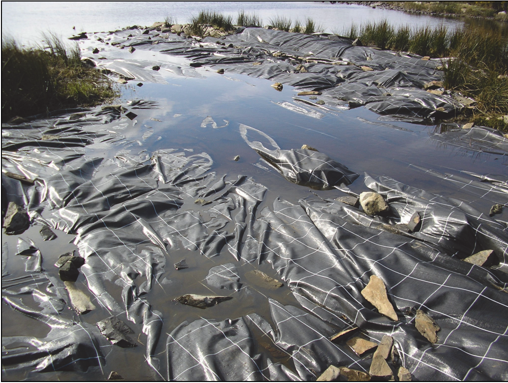
Plate 7. Weed control fabric in place
