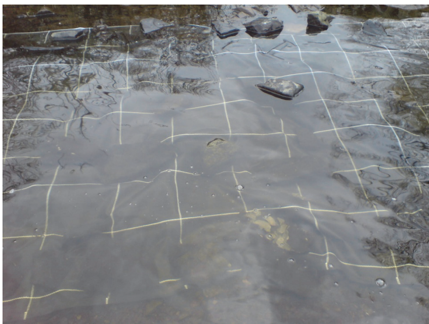
Plate 9. Weighting the join between two lengths of fabric
