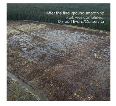
Ground smoothing involved the flipping over, digging in and tracking over of the tree stumps and scrub using low ground pressure excavators to flatten the site and stop the site from drying out. It took two digger drivers around four months each year over the three years to complete the work. This dealt with both issues at Moss of Cree at once.
