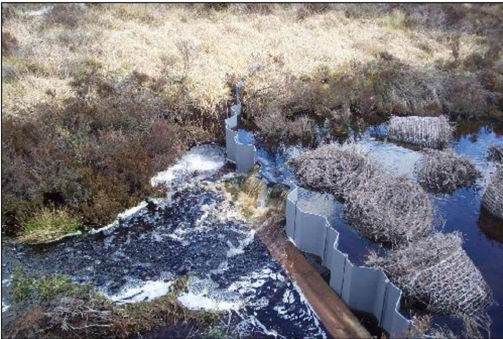
Dam showing support: note that the support is sunk into the ground to enhance stability.
