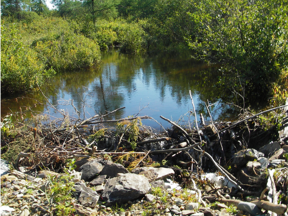
(b) Blocked culvert outflow
