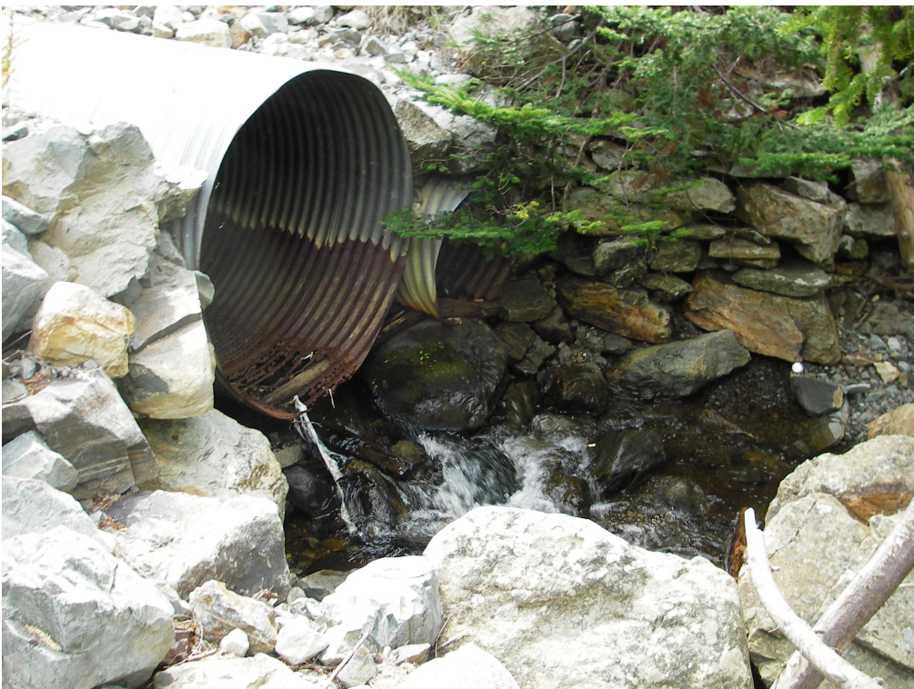
(b) Blocked culvert outflow
