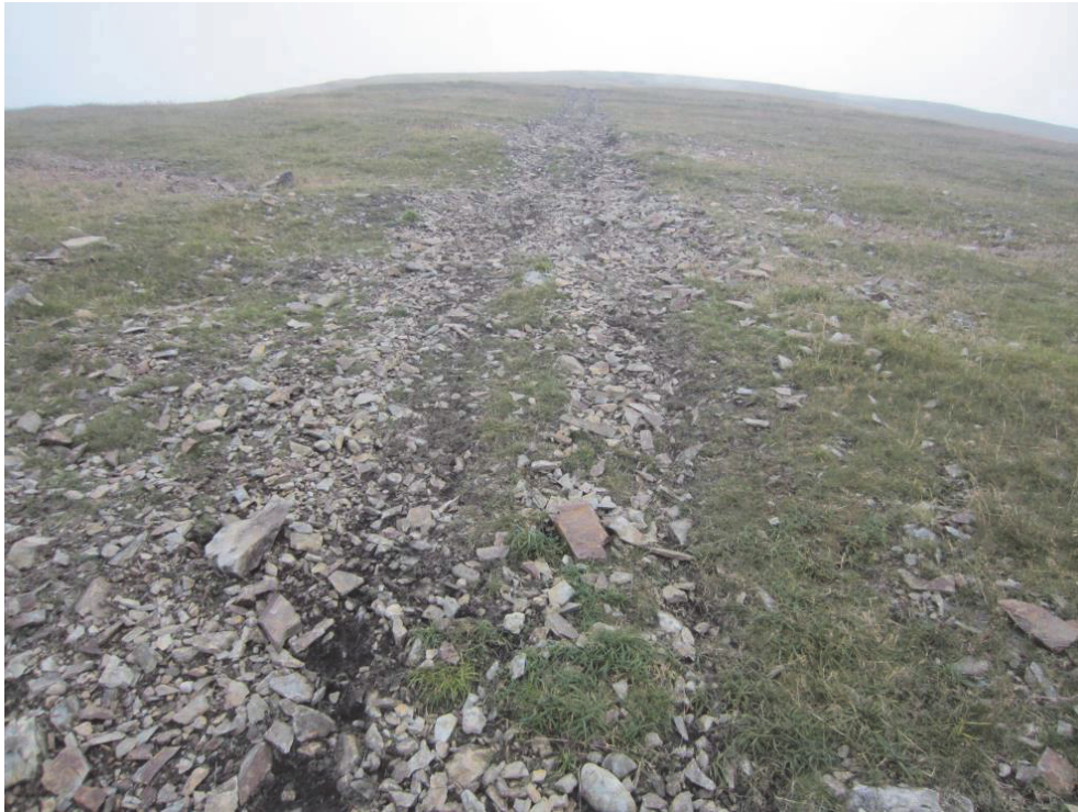
Photograph 149. Vehicle damage high up on the ridge in the east of the site, between Corserine and Carlin's Cairn.
