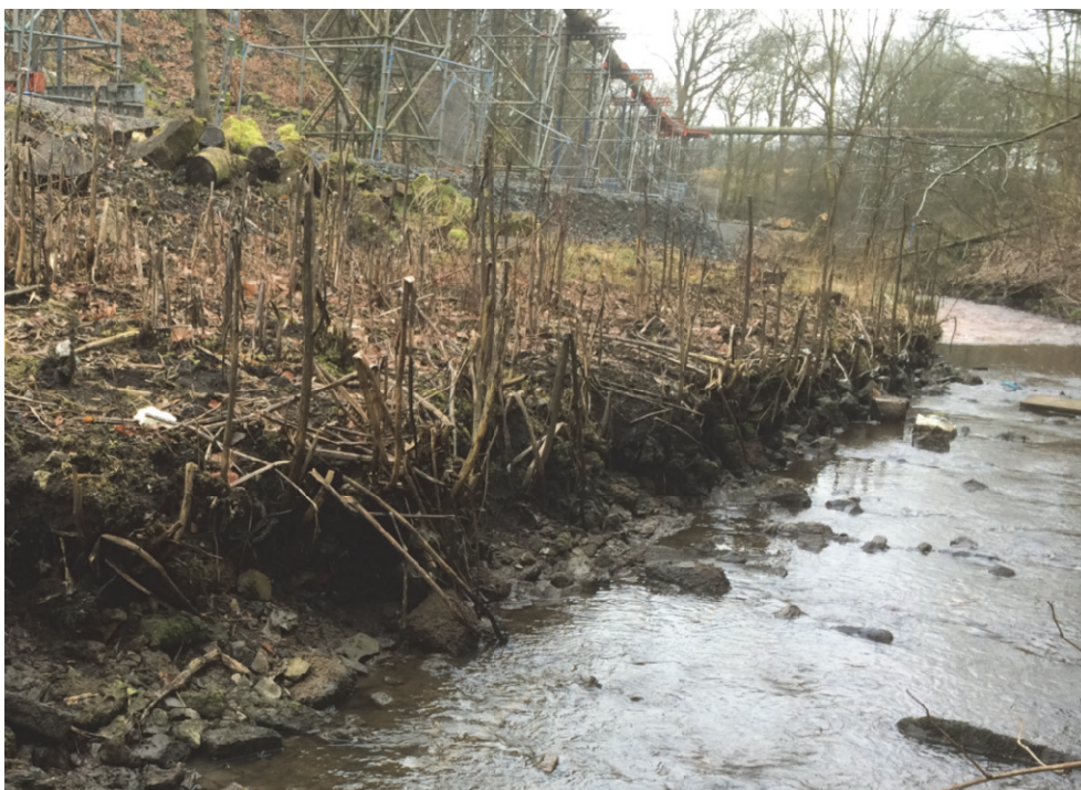
Figure 15. Bank erosion associated with Japanese knotweed.
