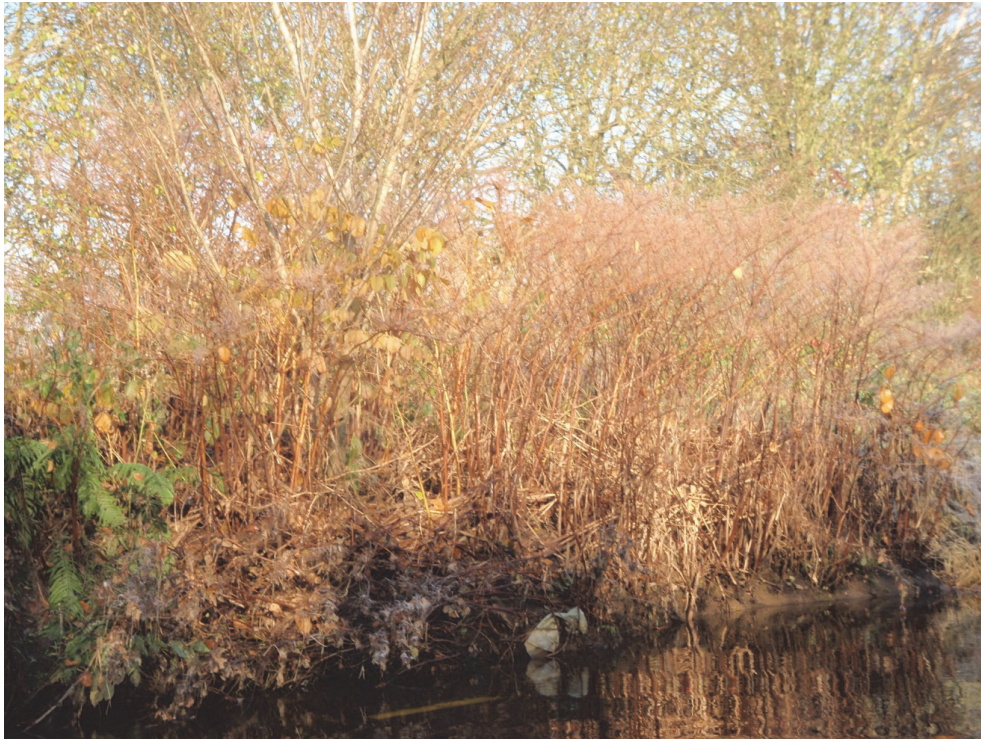
Figure 16. Bank erosion associated with Japanese knotweed.
