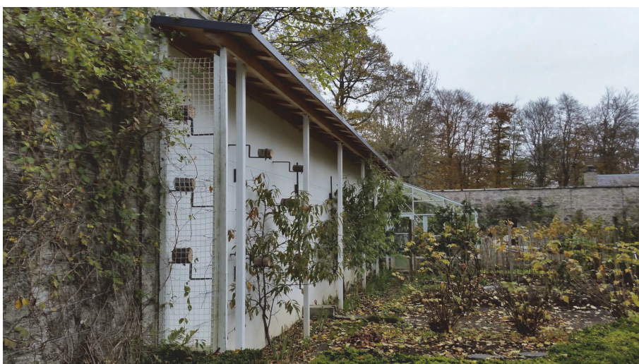
Photograph 36. Example of a contemporary peach pelmet. This helps prevent leaf curl in walled trained trees by reducing the amount of moisture on leaves.
