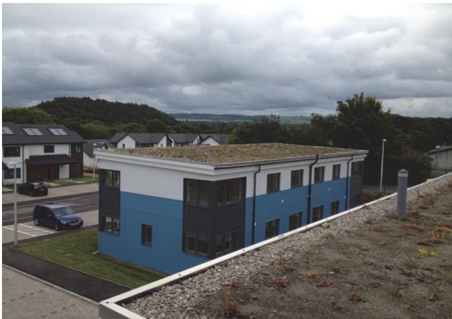
Figure 3. Green roofs on social housing in Inverness (image credit: Caledonia Housing Association).
