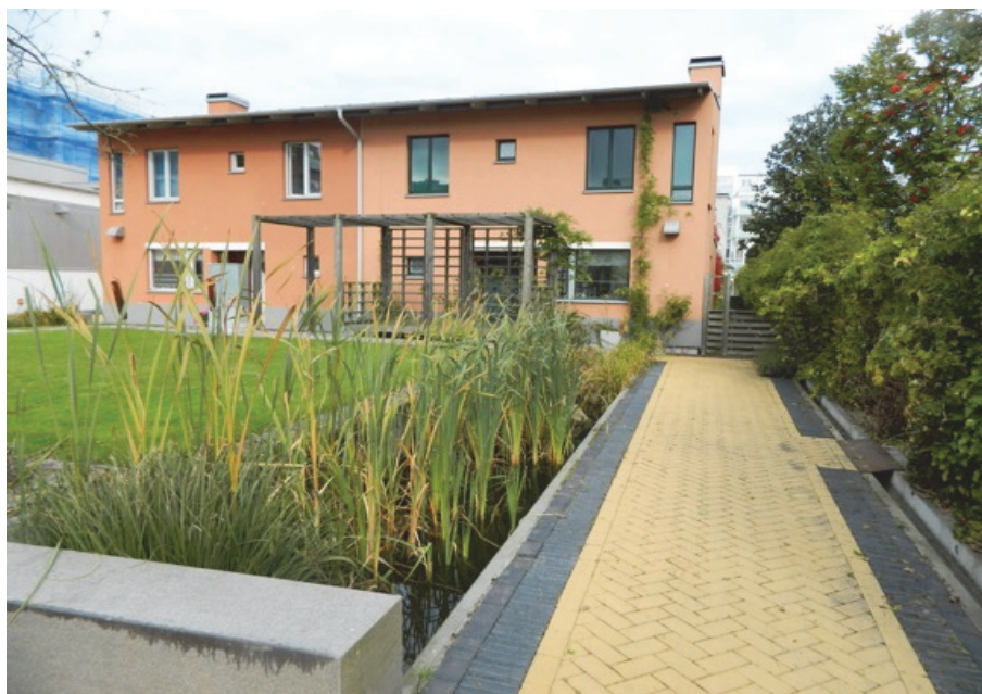
Figure 1. A raingarden in social housing in Malmo, Sweden (image credit: SNH)
