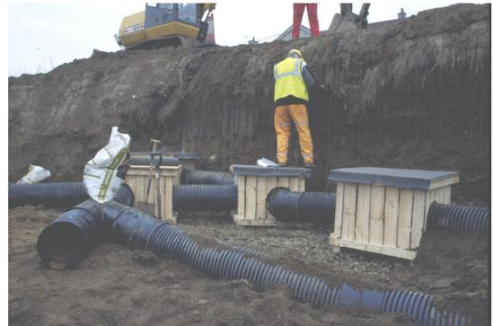
Above: plan of a medium size Type 1 Design artificial sett. Right: Type 1 Design artificial sett under construction, A97, Aberchirder, Scotland (Grampian Badger Surveys for Aberdeenshire Council 2000).
