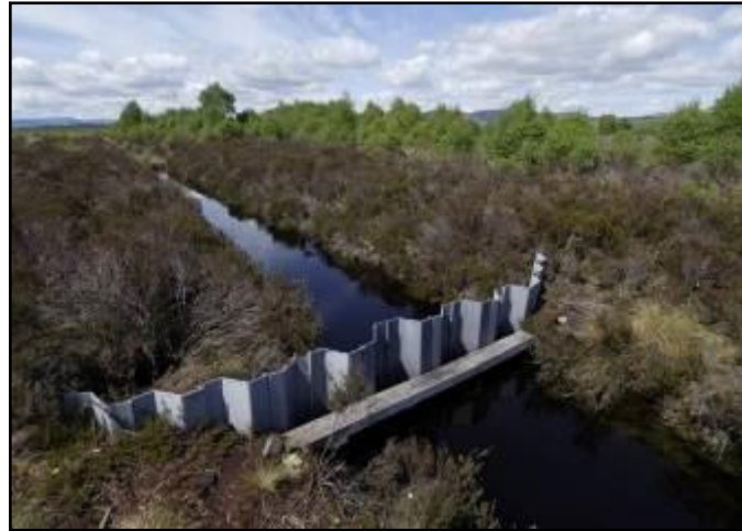
Sheet piling damming a ditch at Flanders Moss
