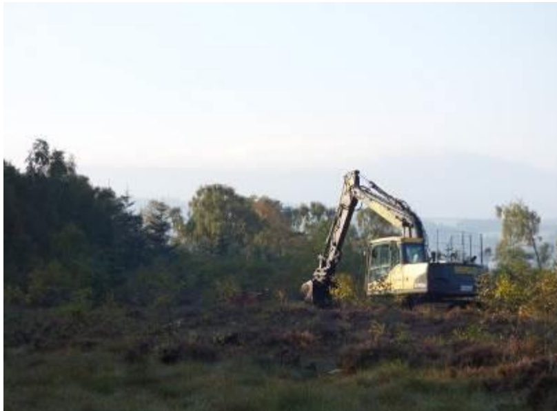
Habitat restoration at Flanders Moss
