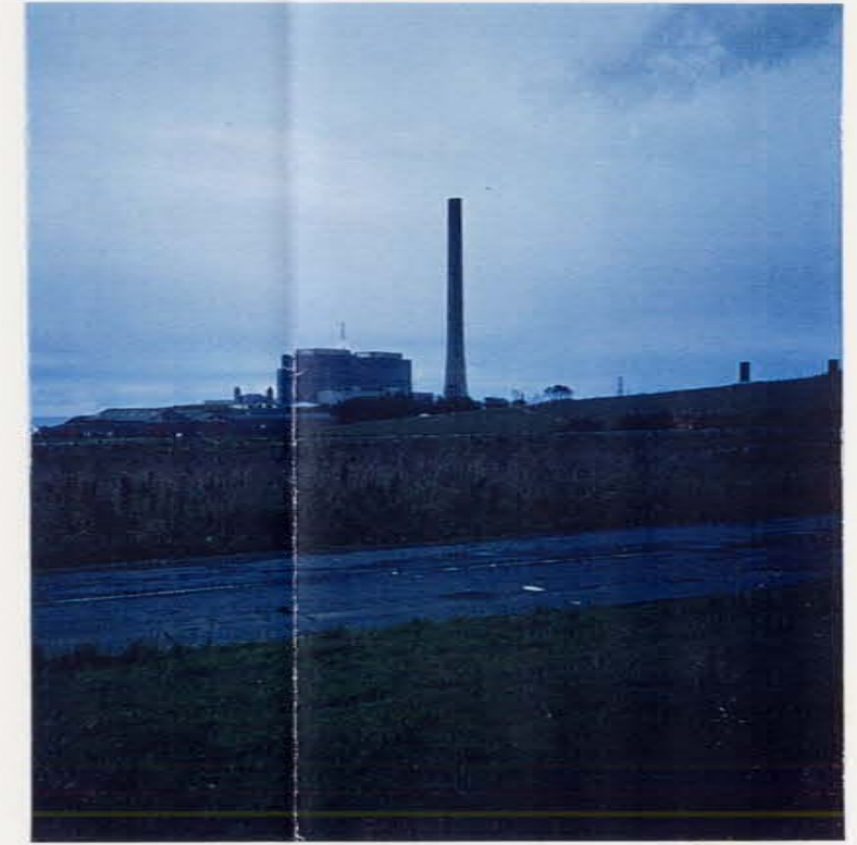
Peterhead Power Station
