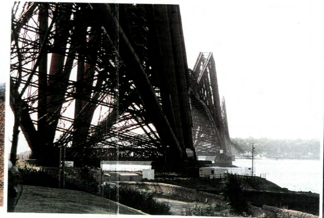
Sub area 39 Firth of Forth (NGR 132 803) - View of the Forth Bridge, from North Queensferry, which has carried trains across the Firth of Forth, at a height of 45 metres, since it was officially opened in 1890, painting of the 45 acres of steel surfaces is still on-going. This stretch of the Firth of Forth, between North and South Queensferry, is totally dominated by the massive structures of both this bridge (Scotland's biggest "listed building") and the Forth Road Bridge.
