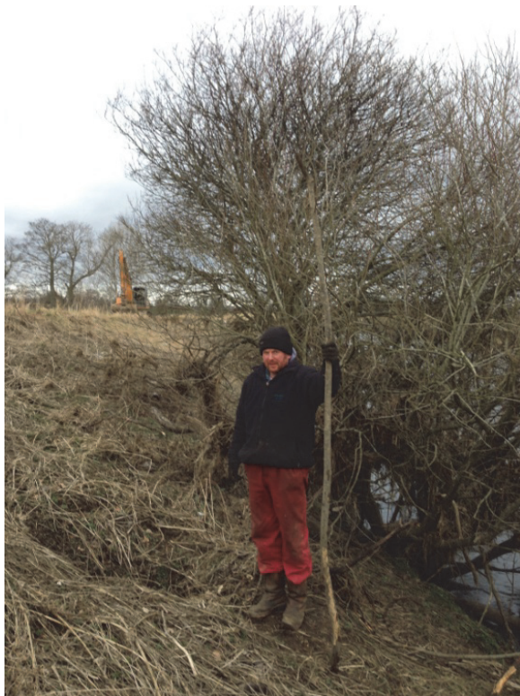
The depth of the blow hole is 3 metres
