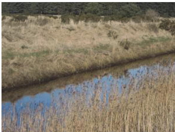
Plate 40. The Spynie Canal to the northwest of the Loch
