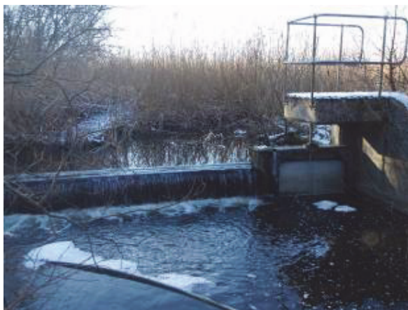
Plate 42. Outflow controlled by weir and sluice
