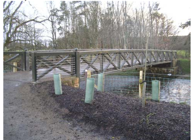
The cycle path now follows a new route via a purpose-built bridge over the Fruin Water, remote from the main road
