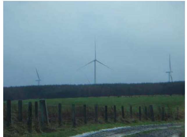
The view of Whitelee Windfarm from an access track to the north
