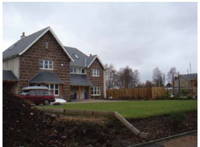
The new housing development
