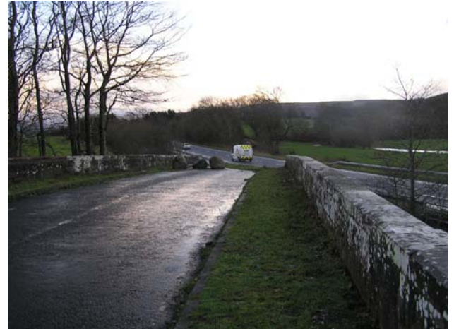
The old route of the cycle path crossed the Fruin Water close to the busy main road
